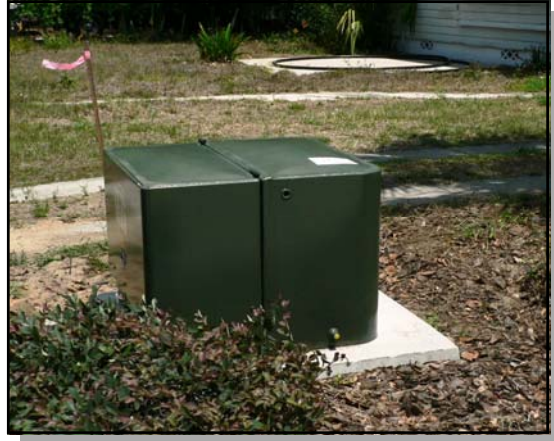
New transformer installation
