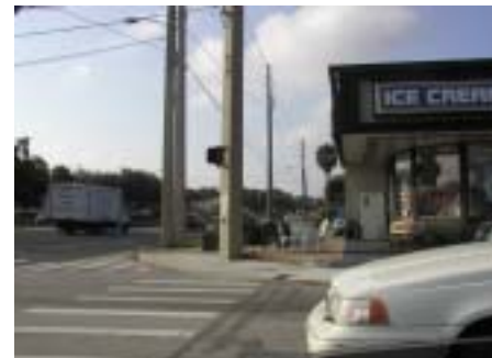
Overhead Utility lines contribute to visual clutter
