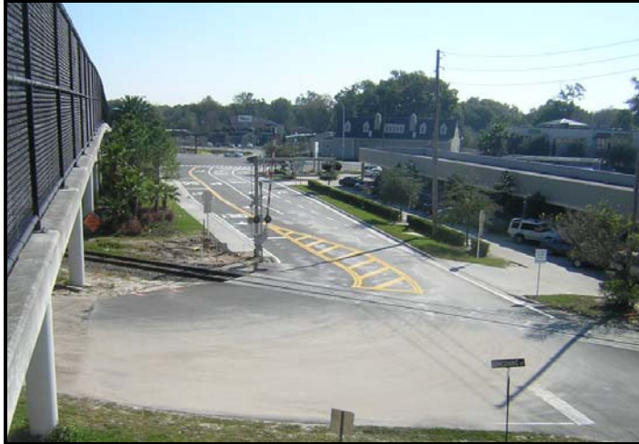
Railroad crossing on Greenwood Road looking east
