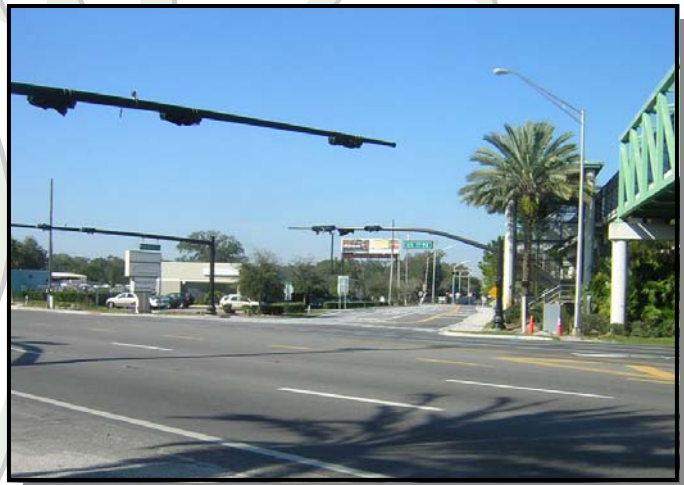
Decorative mast arm poles
