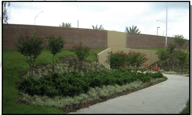
Bike/Pedestrian underpass looking northeast
