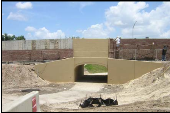
Bike/Pedestrian underpass looking northeast
