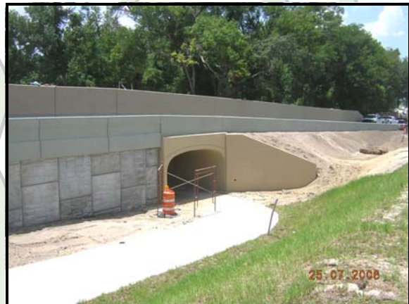
Bike/Pedestrian underpass looking southwest
